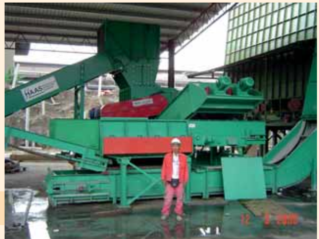
Montage einer Recycling-Anlage in Sarawak (Borneo/Kalimantan).
